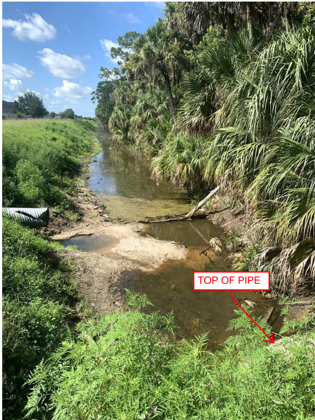
South End of Pipe (top view)
