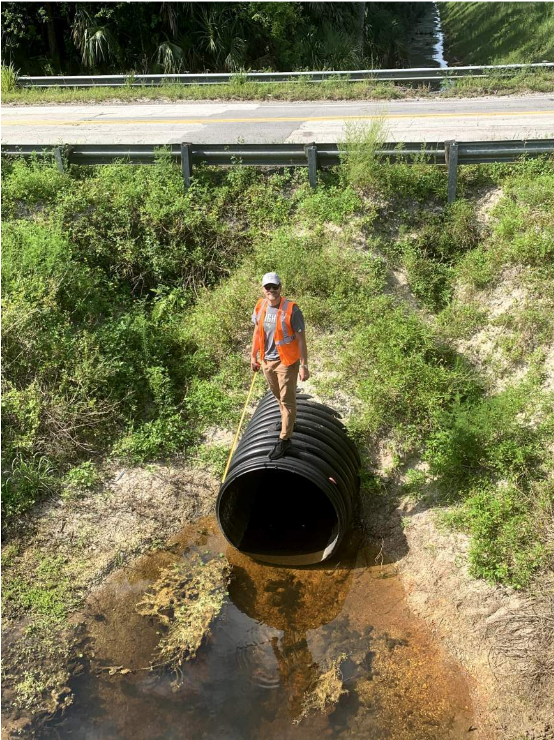
North End of Pipe
