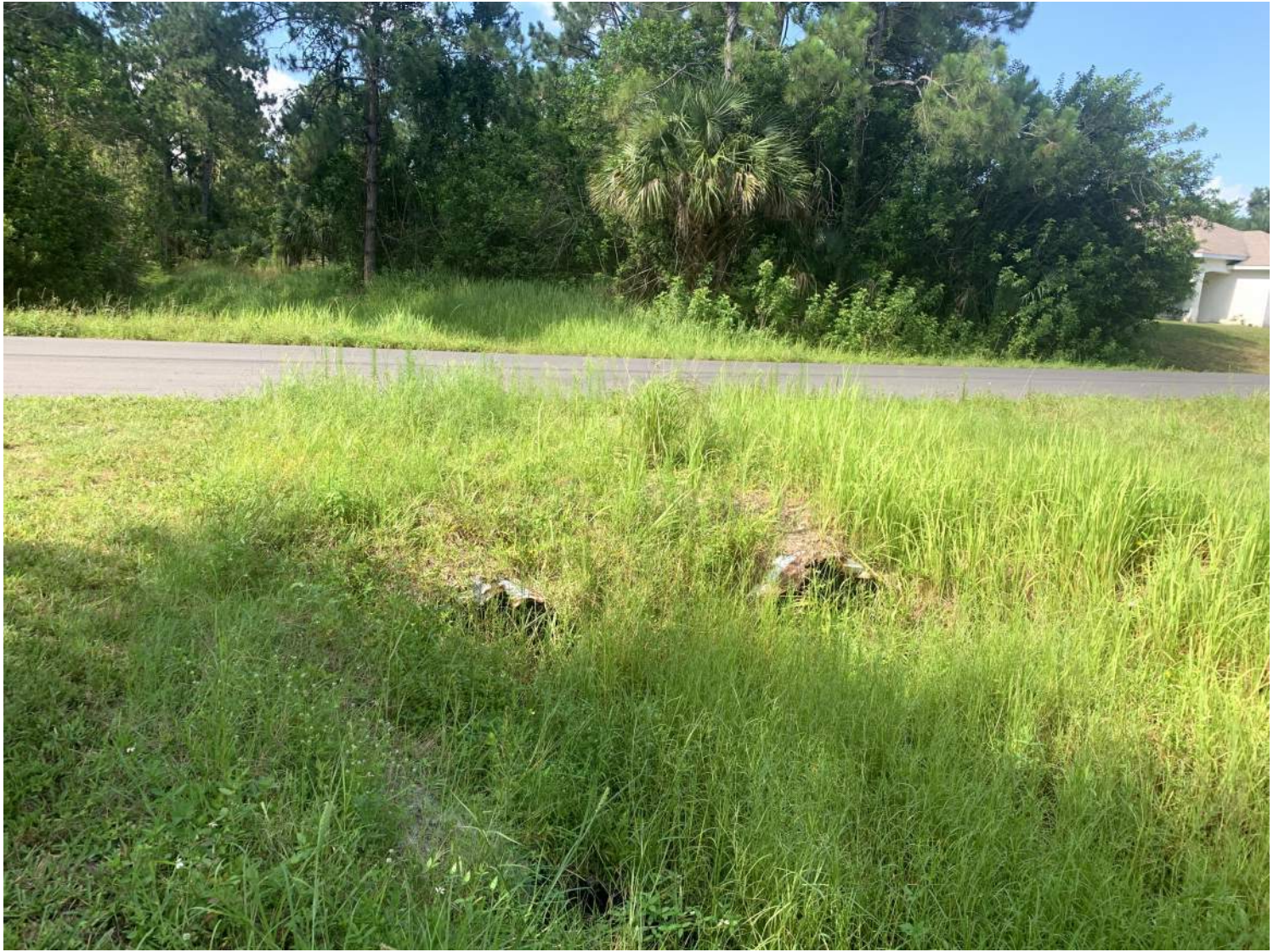
South End of Pipe
