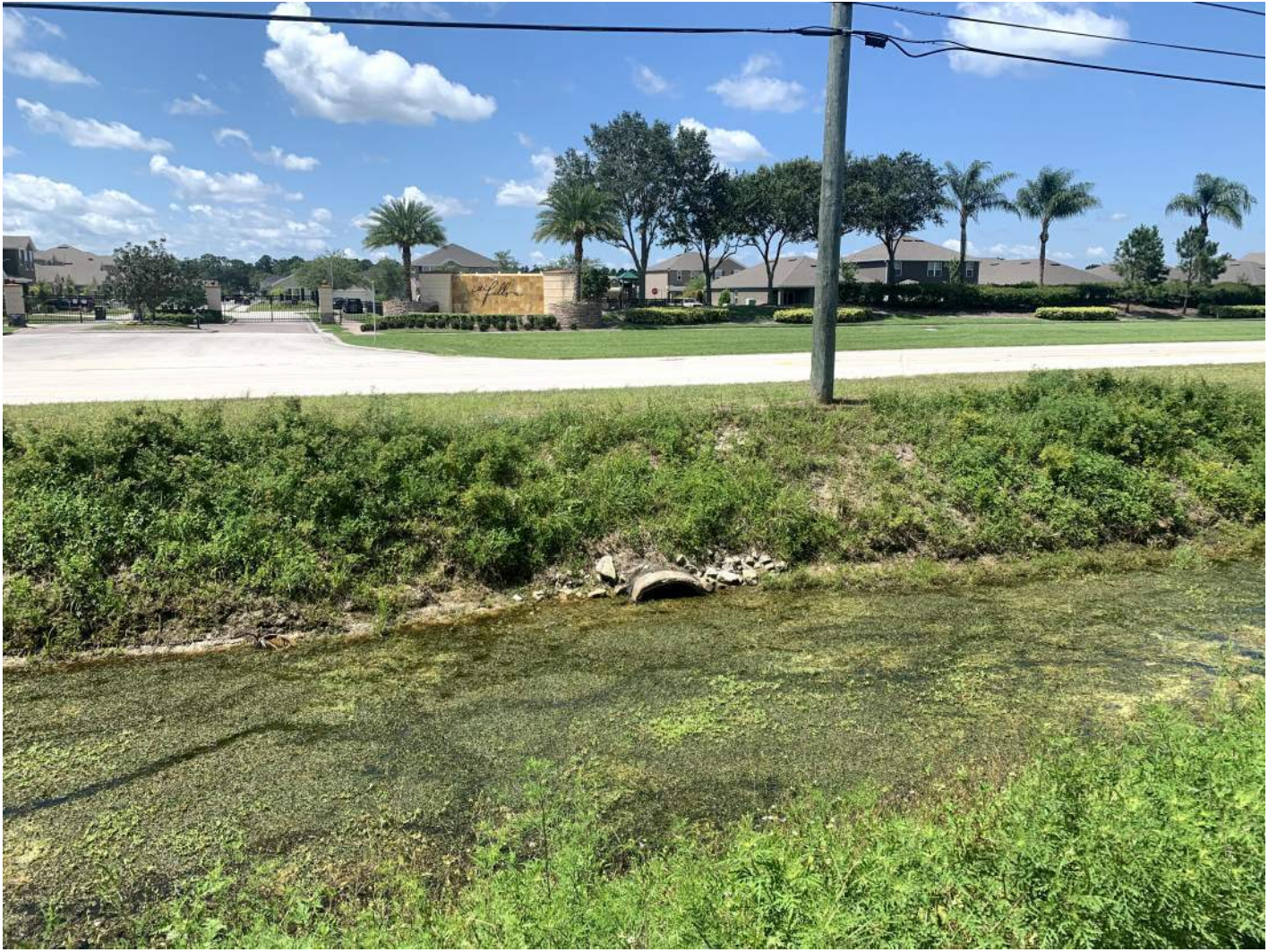
North End of Pipe
