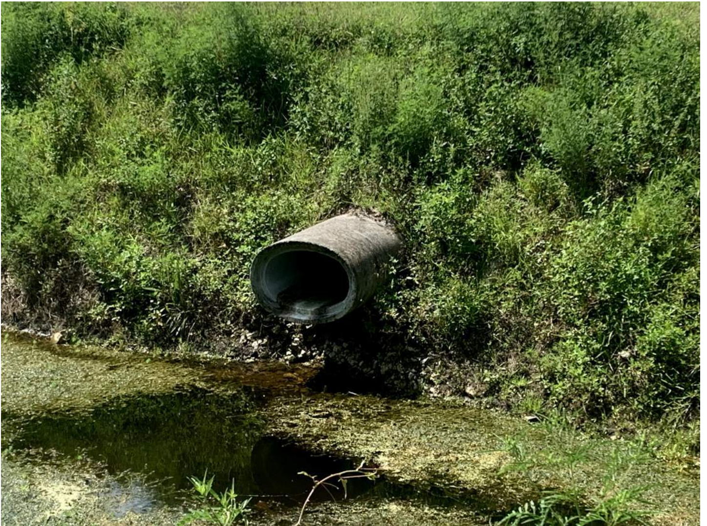
North End of Pipe
