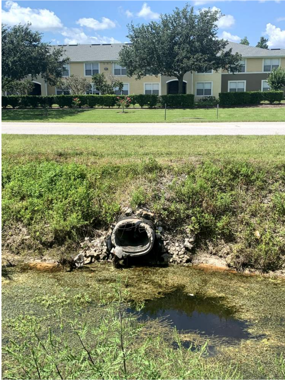
North End of Pipe
