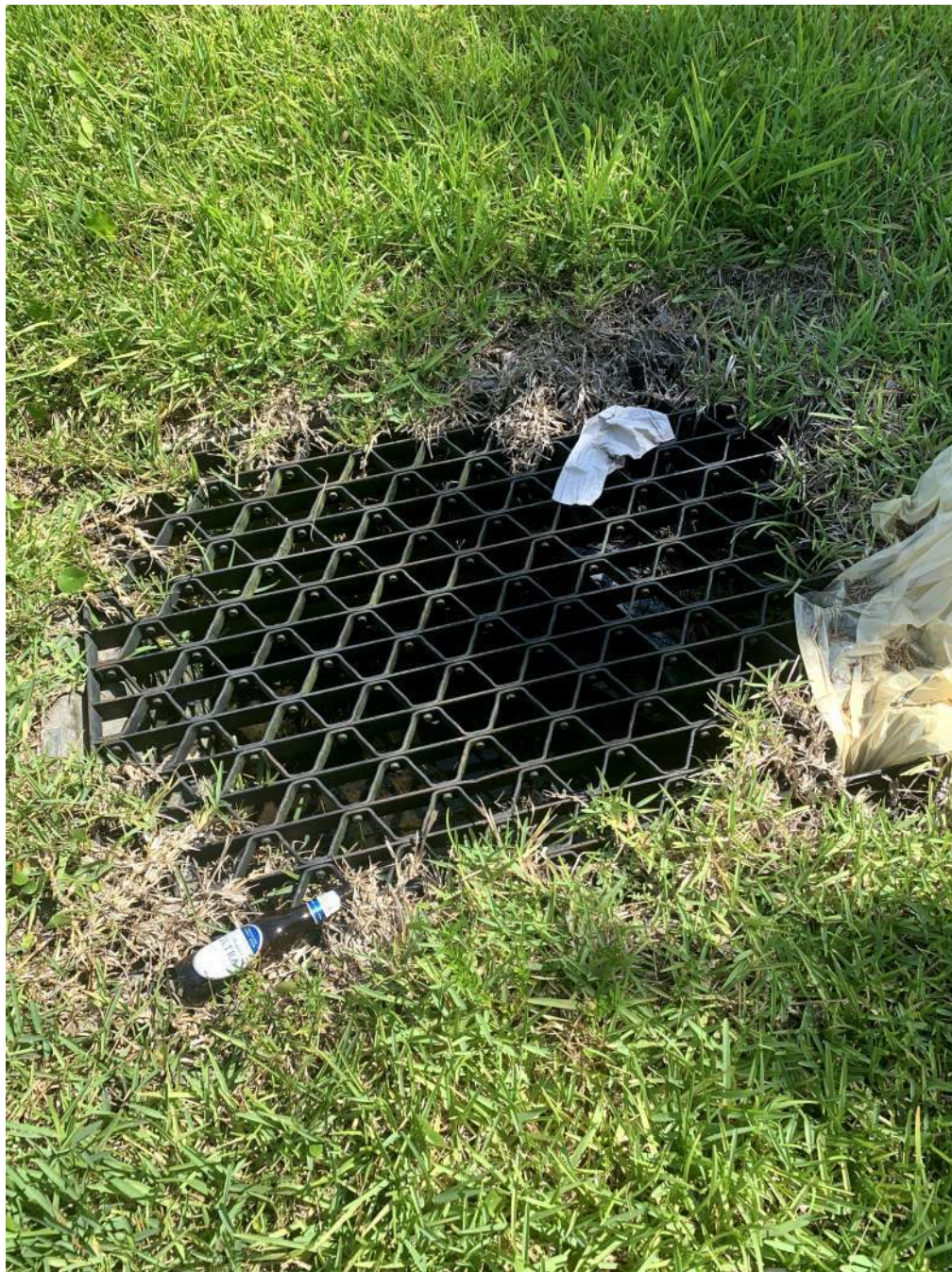
South Catch Basin
