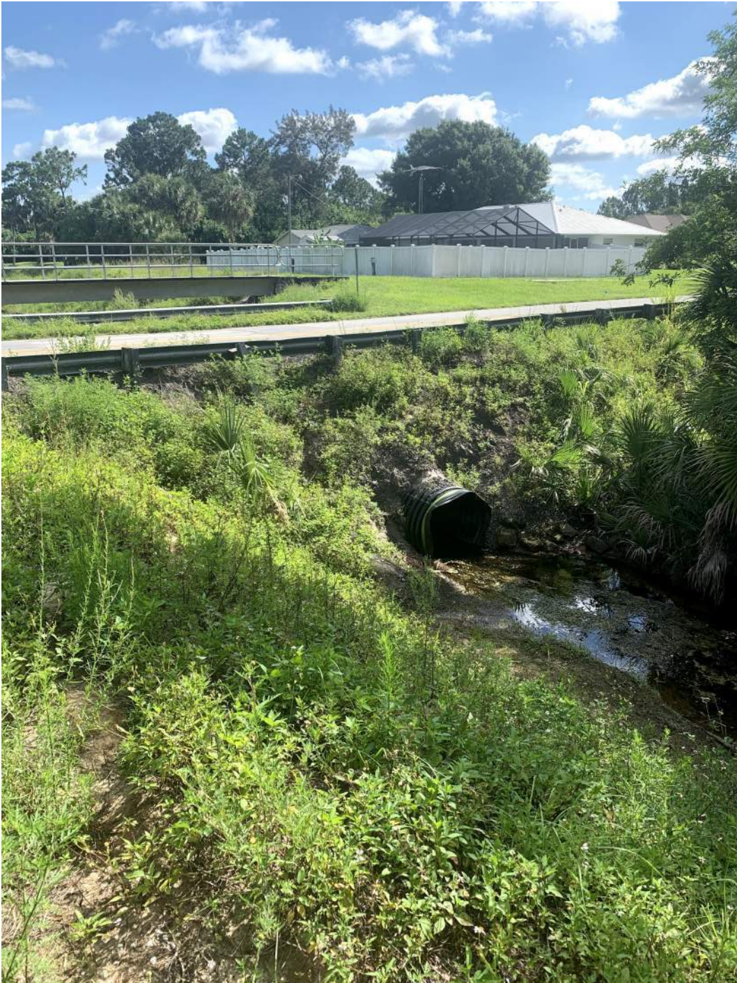
South End of Pipe
